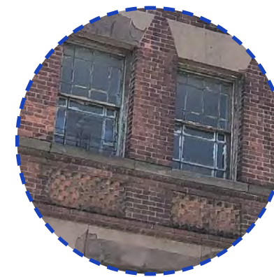
TEXTURED BRICK COURSING
